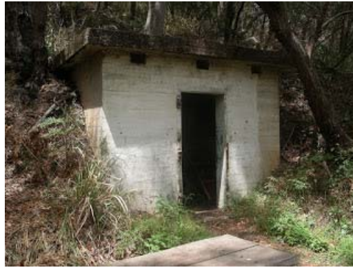
Concrete utility room on Tomaree Headland
