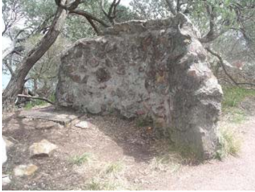
Remains of a rock structure on the summit. During the war years buildings at the Radar Station were camouflaged, by mesh and cement to make them appear like rocks
